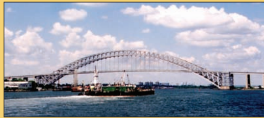
The Bayonne Bridge on the Kill van Kull.
